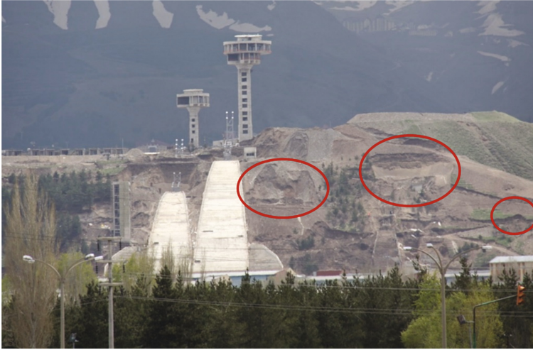
Fig. 6. Local slope failures in the field during construction
