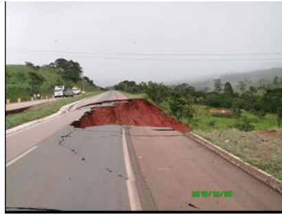
Fig. 6. Broken section of the BR-060/GO (12/30/2010).
