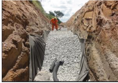
Fig. 17. Execution of deep drains.
