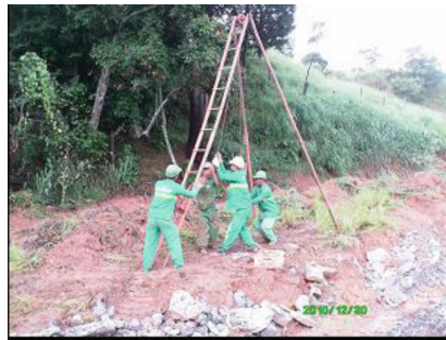
Fig. 12. Execution view of the SPT 1 survey (BR-060, km 24).
