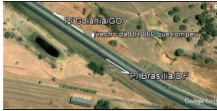
Fig. 2. Broken section of BR-060/GO (12/31/2010).
