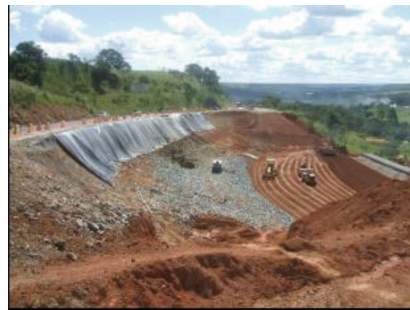
Fig. 19. Execution of the draining mattress.
