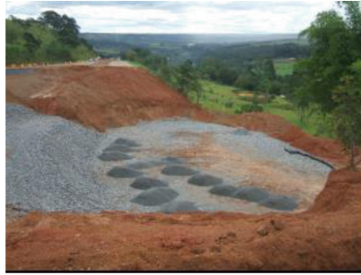
Fig. 20. Drainage mattress construction.
