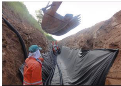
Fig. 16. Execution of deep drains.
