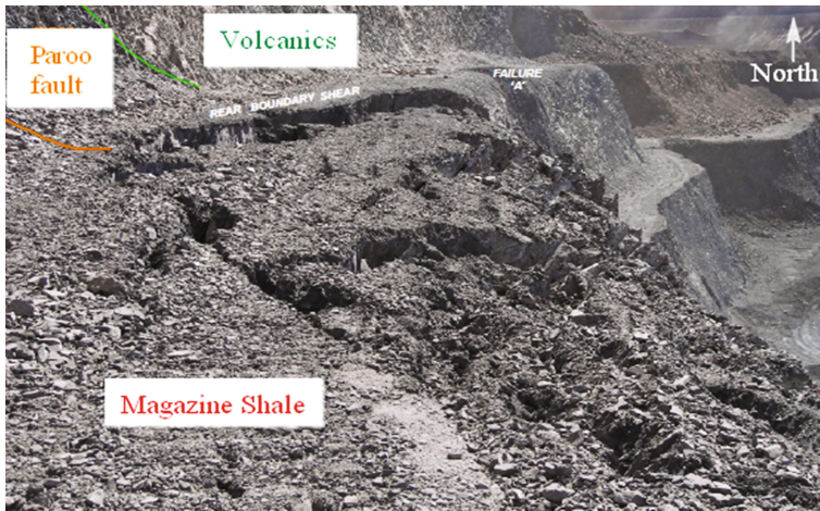
Fig. 9. Top of failure on RL3,400, July 17, 2008, looking north (after Rosengren and Associates 2008)
