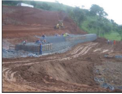
Fig. 24. Execution of gabion restraint.
