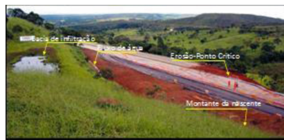
Fig. 9. Infiltration basin upstream of the highway (Lino 2016).
