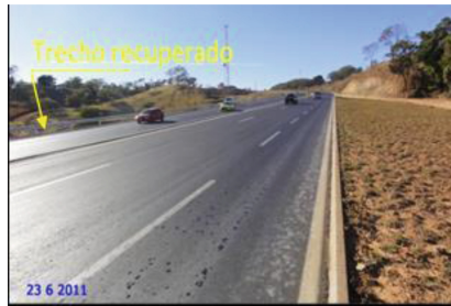
Fig. 28. Retrieved and completed section.
