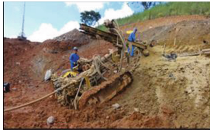
Fig. 18. Drilling for DHP installation.
