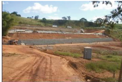
Fig. 26. View of gabion restraint.
