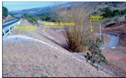
Fig. 21. Smooth waterfall running along the banks of the stretch recovered on Highway BR 060.
