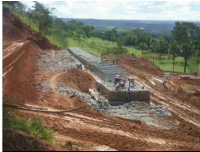
Fig. 25. Execution of gabion restraint.
