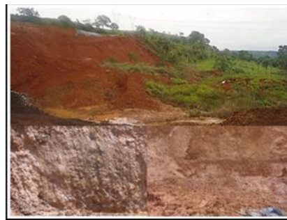
Fig. 10. View of saturated soil after landslide, December 2010 (Lino 2016).
