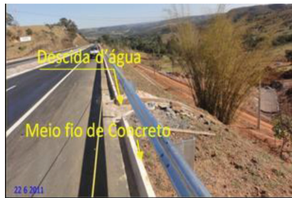
Fig. 29. Retrieved and completed section.
