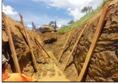
Fig. 15. Excavations for the installation of deep drains.
